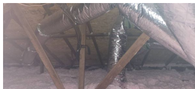
Bracing is not properly supported
